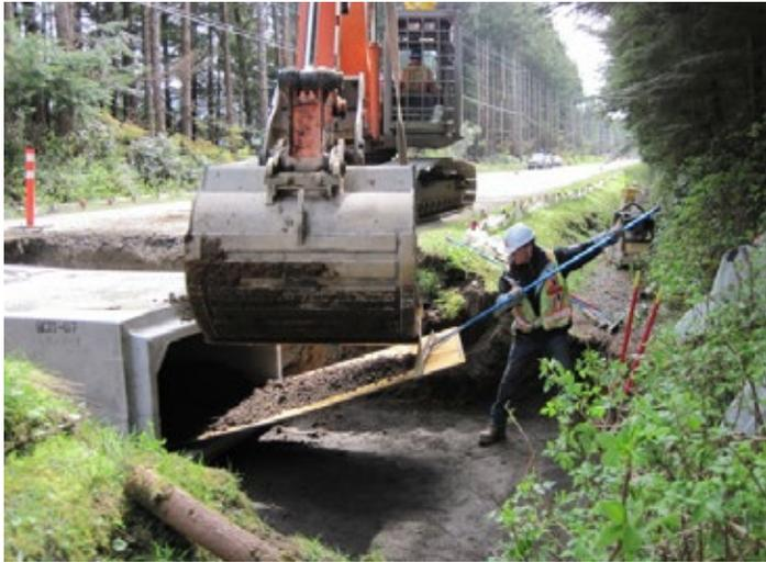
Fig. 3: Installation of a pre-fabricated concrete box culvert. Photo: Barbara Beasley.
